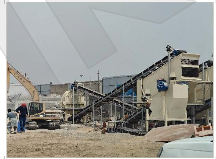
CRUSHING AND SCREENING PLANT, RAS AL KHOR
