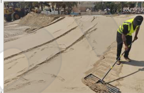
— FINAL LEVELLING AND FINISHING
