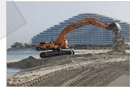
EARTHWORKS AND RECLAMATION
