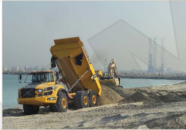
— RECLAMATION AND BREAKWATER WORKS
