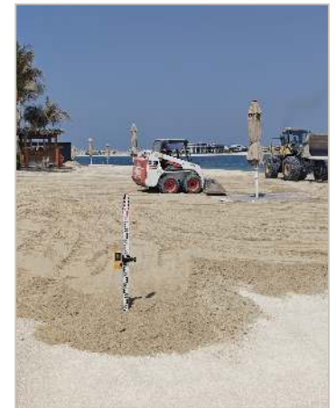
PROFILING TO SURVEY LEVELS
